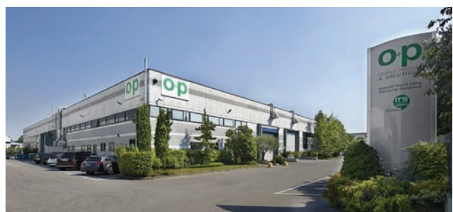
O+P Head Office - Brescia, Italy
